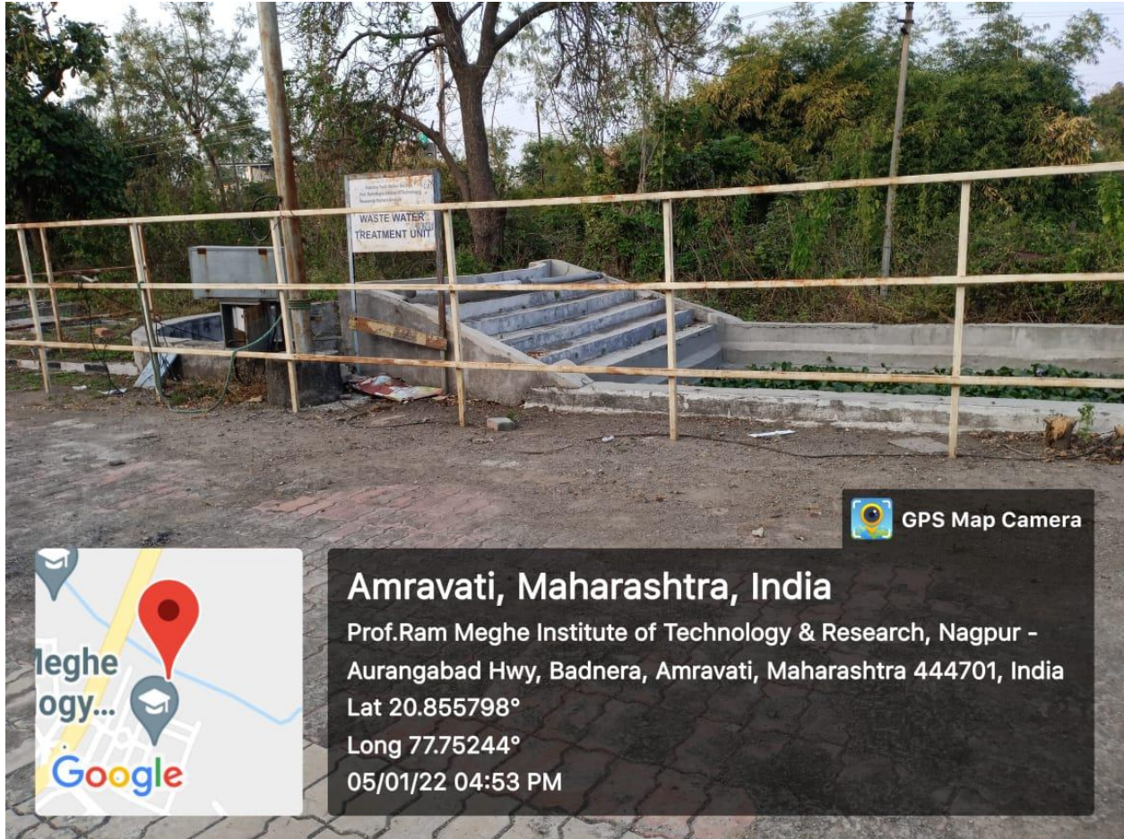
Waste water recycle
