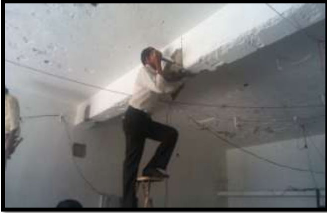
Rebound Hammer test
